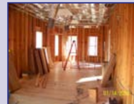
Construction at Bible Baptist Church
